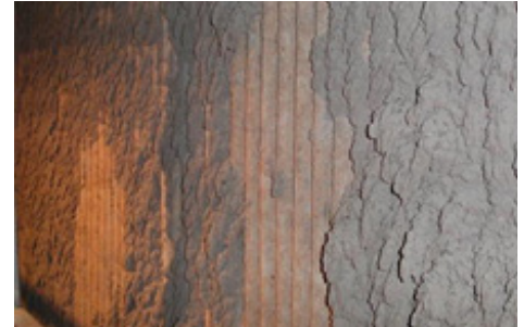
Figure 2: Slag on tubes
